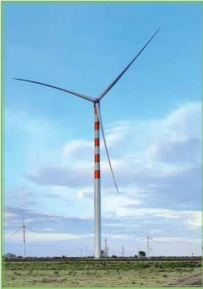
IREDA funded 252 MW Wind Project at Maniyachi site, Tuticorin District, Tamil Nadu
