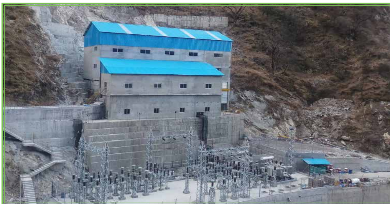
IREDA funded 24 MW Dikshi Hydroelectric Project at West Kameng, Arunachal Pradesh.
