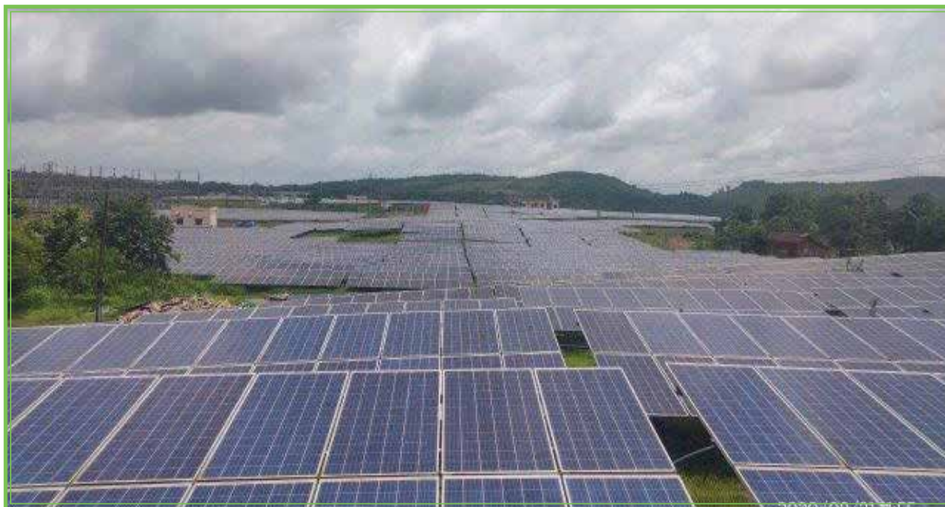
IREDA's 50 MW Solar PV Project at Kasargod, Kerala.
