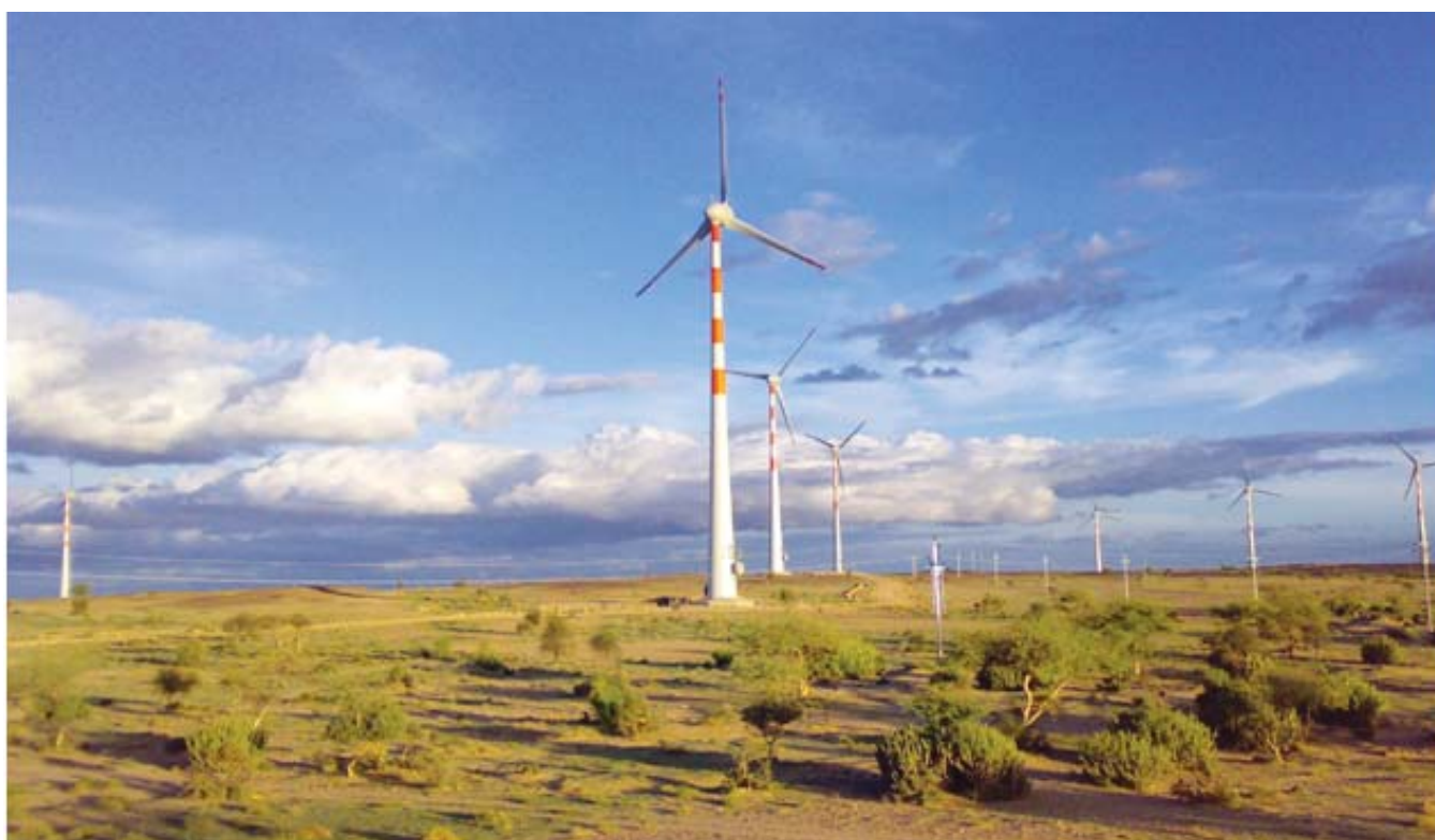
45 MW wind power project set up in the state of Rajasthan
