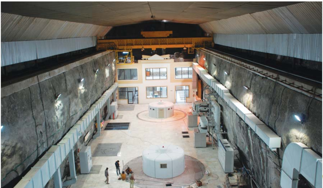
Power House Complex with Unit-1 & 2
