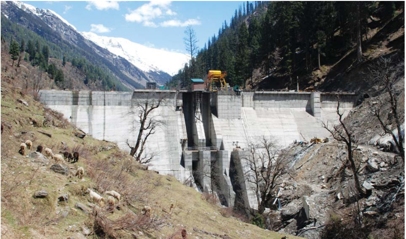
Dam- Down Stream Side view
