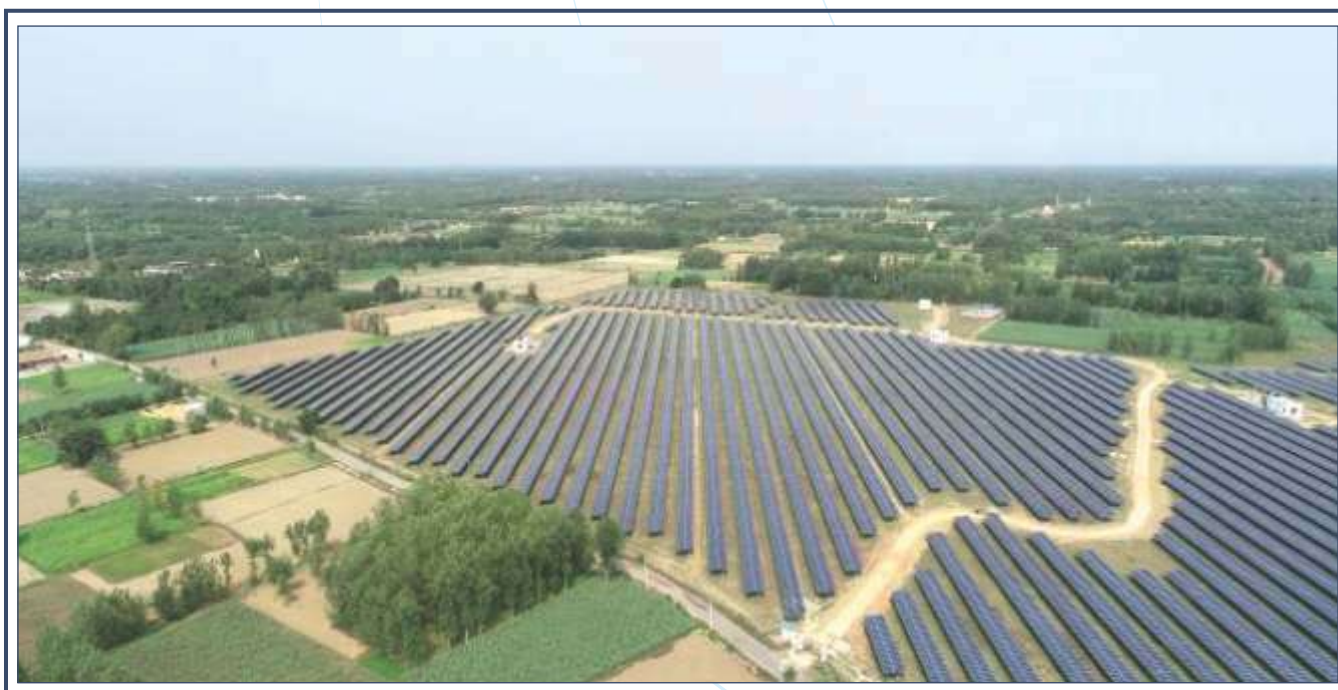
IREDA funded 6 Solar PV projects of EDEN Group situated in Uttarakhand
