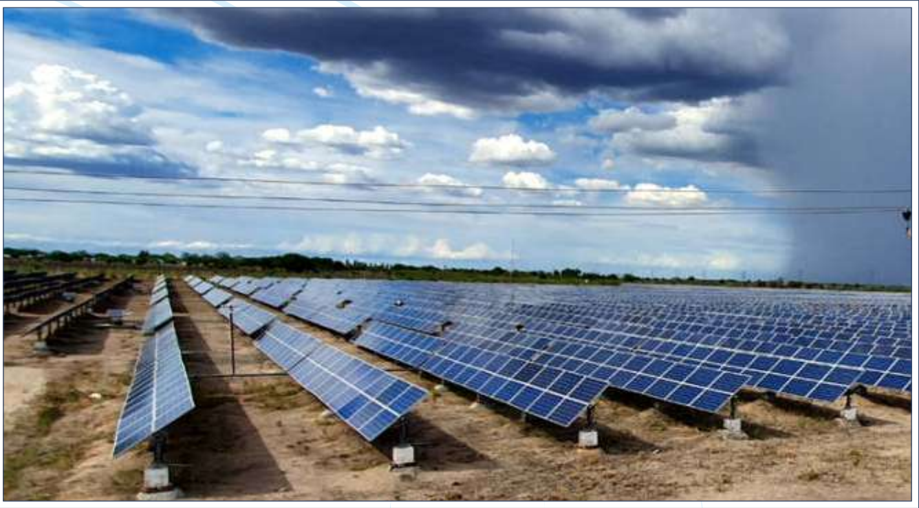
IREDA funded 5 MW Solar PV grid connected project located at Virudanagar District, Tamil Nadu.
