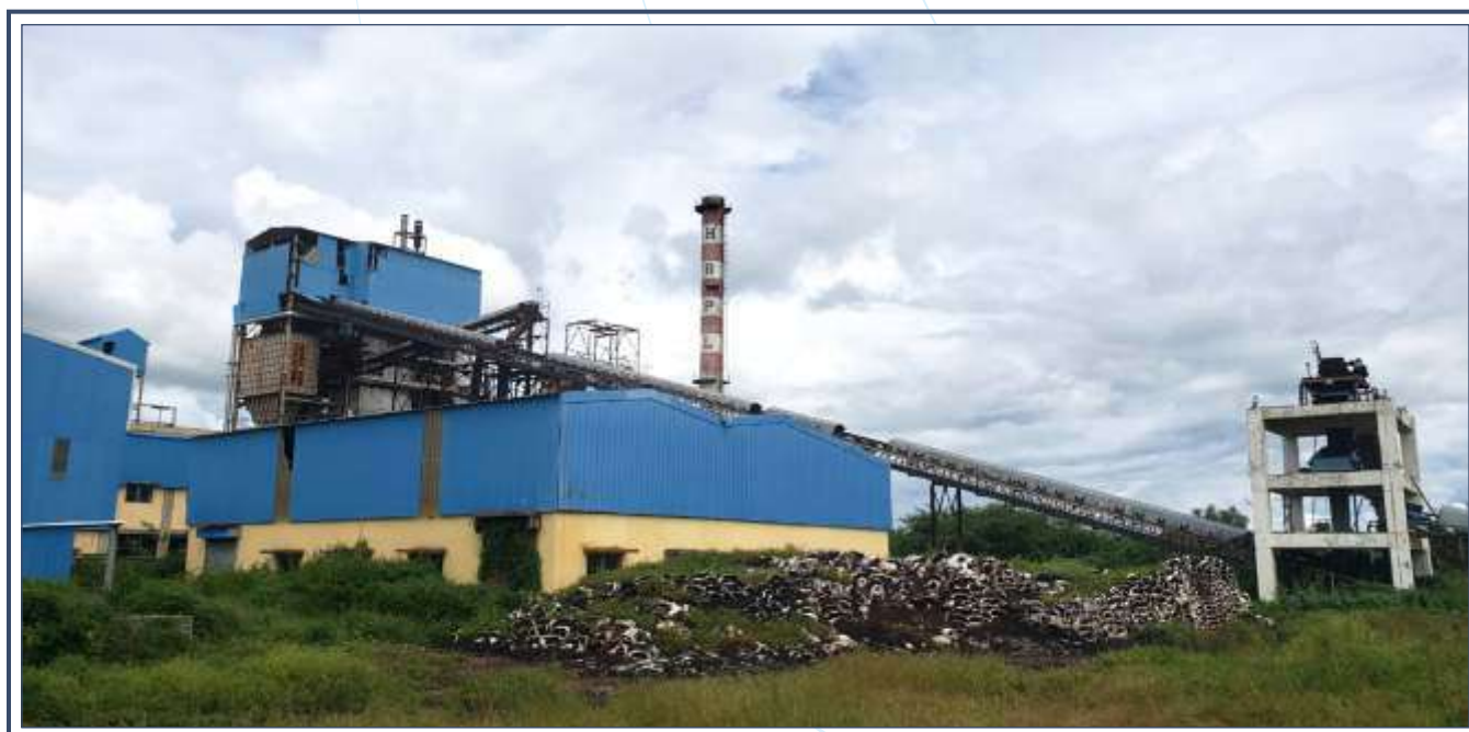
IREDA funded 10 MW Haveri Bioenergy Ltd. Biomass based power plant, Karnataka.
