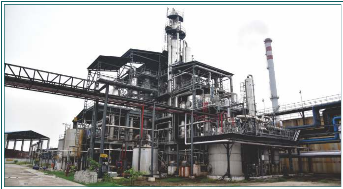
IREDA funded 100 KLPD capacity Ethanol manufacturing Plant of M/s. Gobind Sugar Mills Pvt. Ltd. located at Aira Estate, Lahimpur Kheri, Uttar Pradesh.
