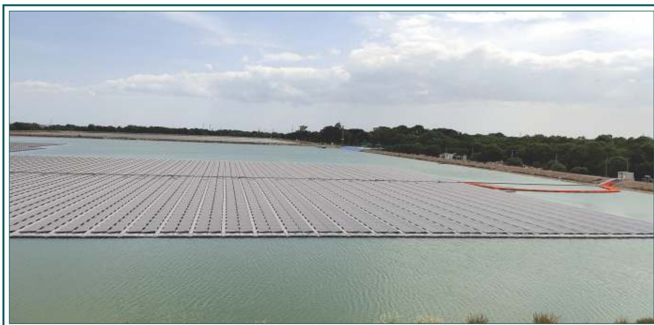
IREDA funded 22 MWac /25.681 MWp Floating Solar PV Plant of M/s Greenam Energy Pvt. Ltd., located at Muthiahpuram village, Thoothukudi District, Tamil Nadu.
