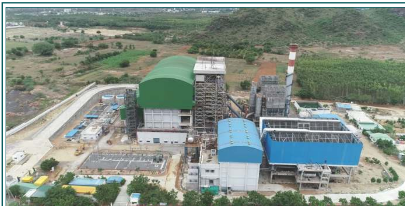
IREDA funded 15 MW Waste to Energy project of M/s. Jindal Urban Waste Management (Guntur) Ltd., located at Kondaveedu village, Edlapadu Mandal, District Guntur, Andhra Pradesh.
