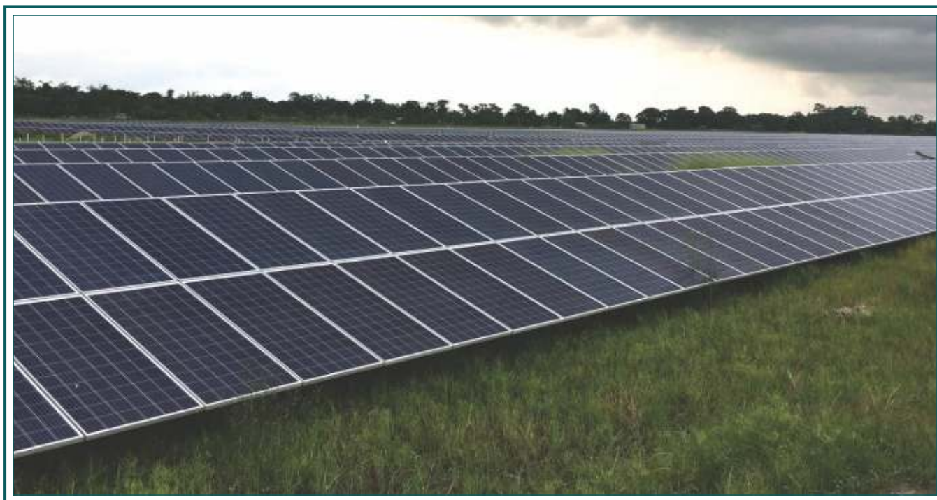
IREDA funded 90 MW Solar PV Power Project of M/s. Azure Power Forty Pvt. Ltd. located at Assam.
