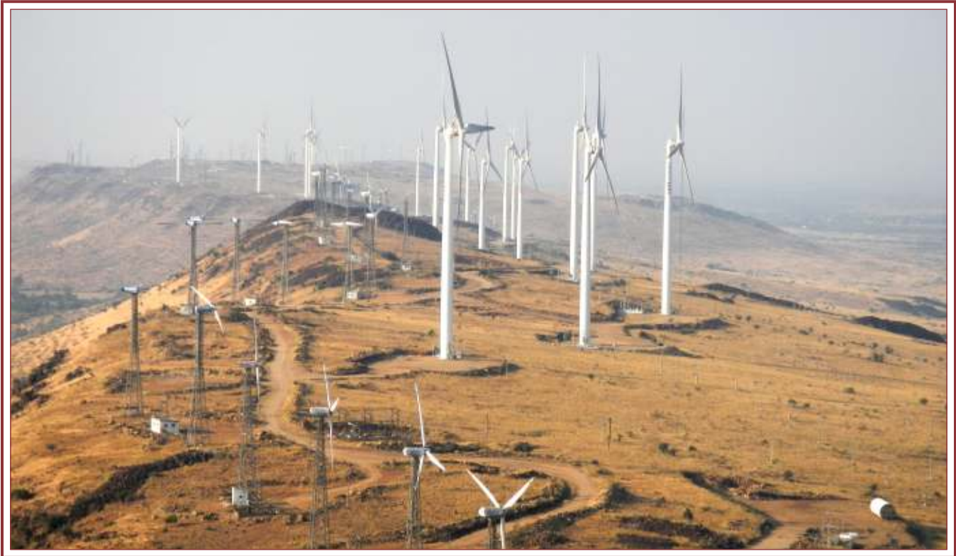
IREDA funded 241 MW Wind Farm Project of M/s. Beta Wind Farm Pvt. Ltd. located at Tadipatri, Ananthapur District, Andhra Pradesh
