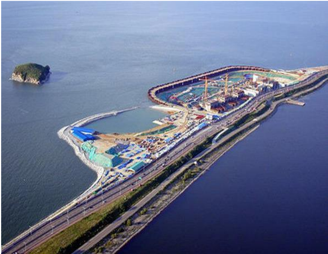
Figure 27: Shiwa Lake Tidal Barrage
