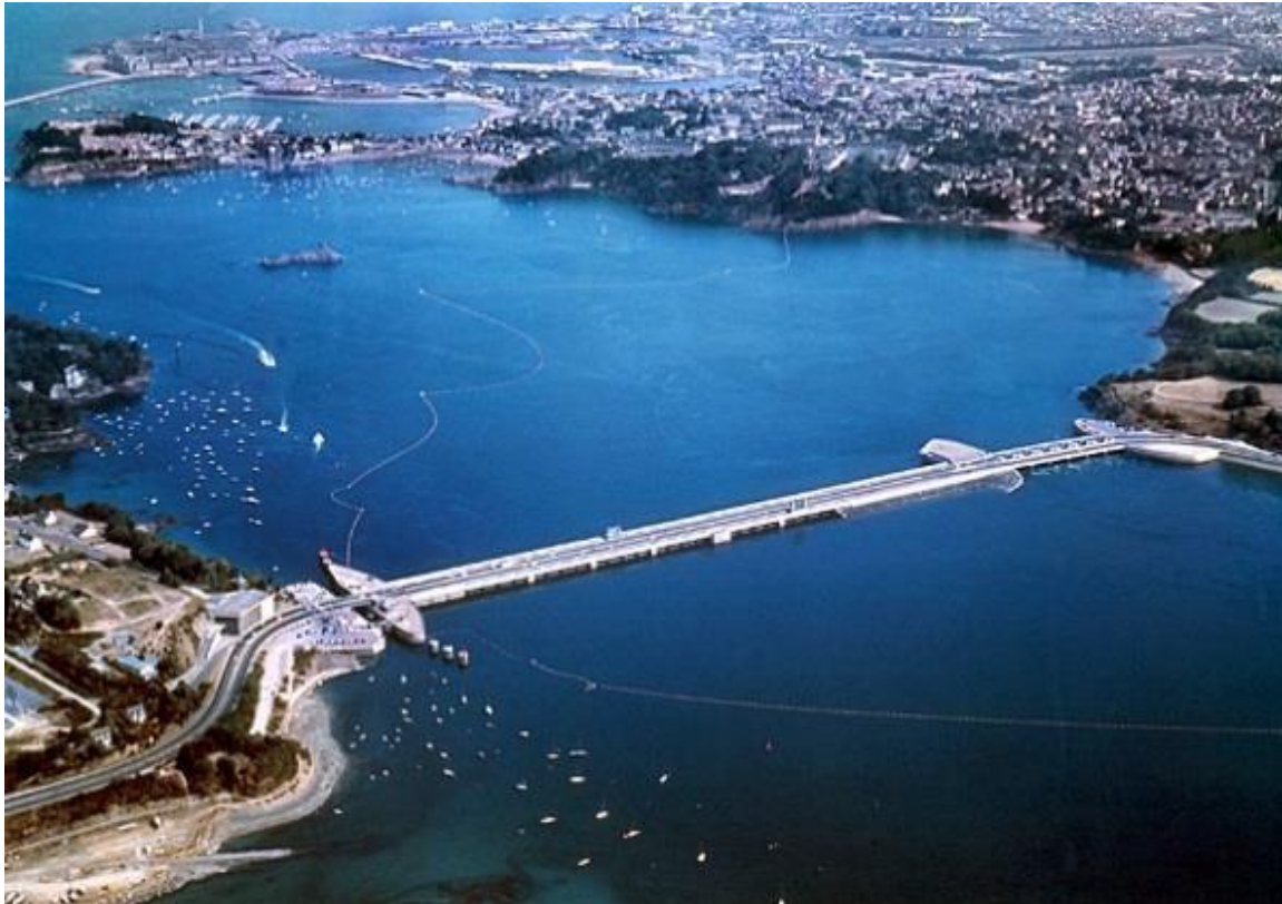
Figure 26: La Rance Tidal Barrage
