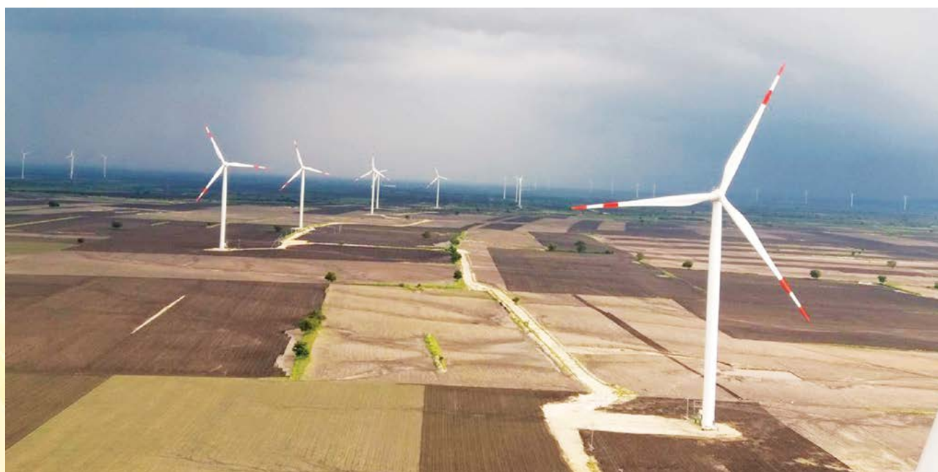
IREDA funded 226.80 MW project in the state of Andhra Pradesh.
