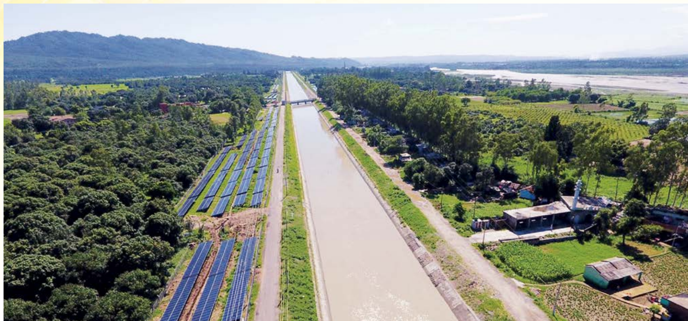
IREDA funded 14.5 MW Canal Bank Solar PV Project in District Dehradun, Uttarakhand
