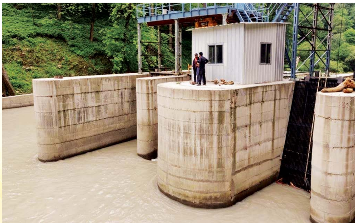
IREDA funded 9.00 MW Balargha Small Hydro Project located at Village Balargha, Tehsil – Phati Manikaran, Dist-Kullu, Himachal Pradesh.
