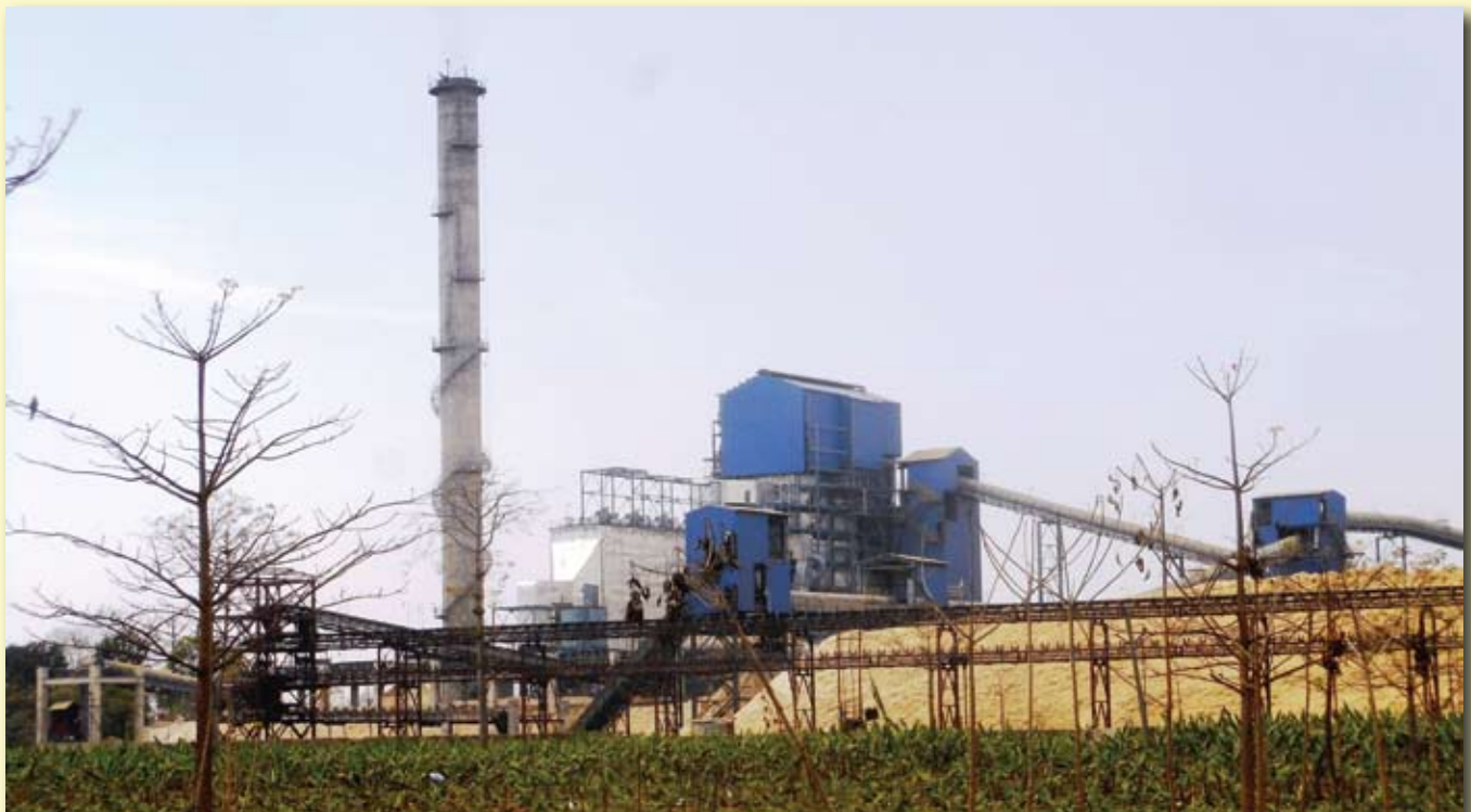
IREDA financed 30 MW Cogeneration Project at Lakhimpur Kheri of Uttar Pradesh
