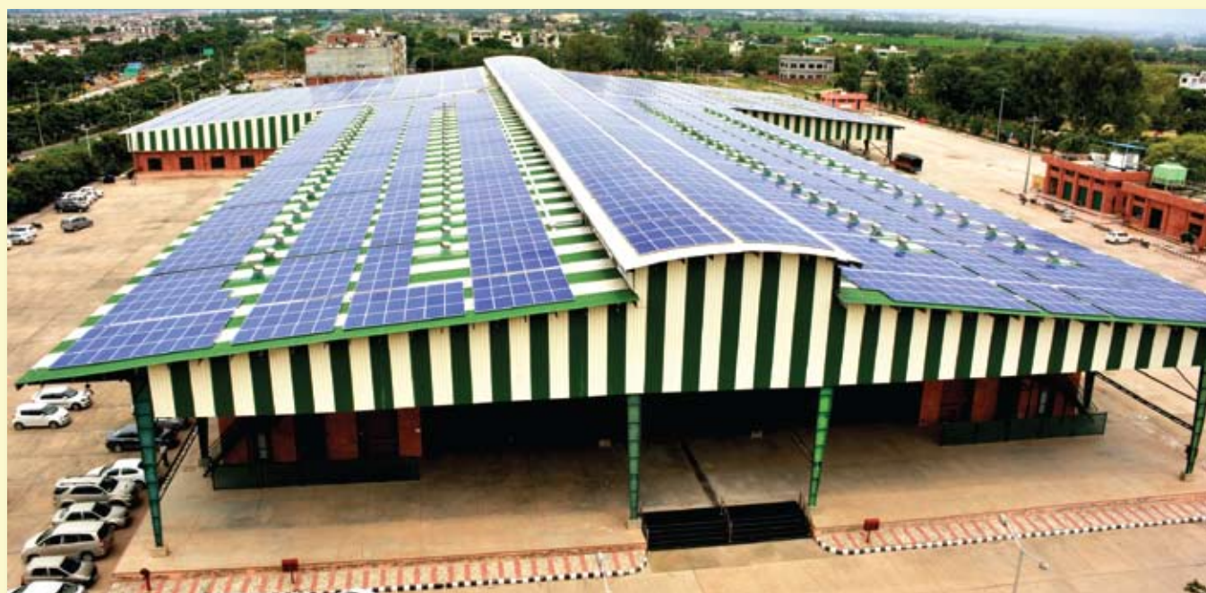
IREDA financed 10MW Solar PV Rooftop Plant at Punjab.
