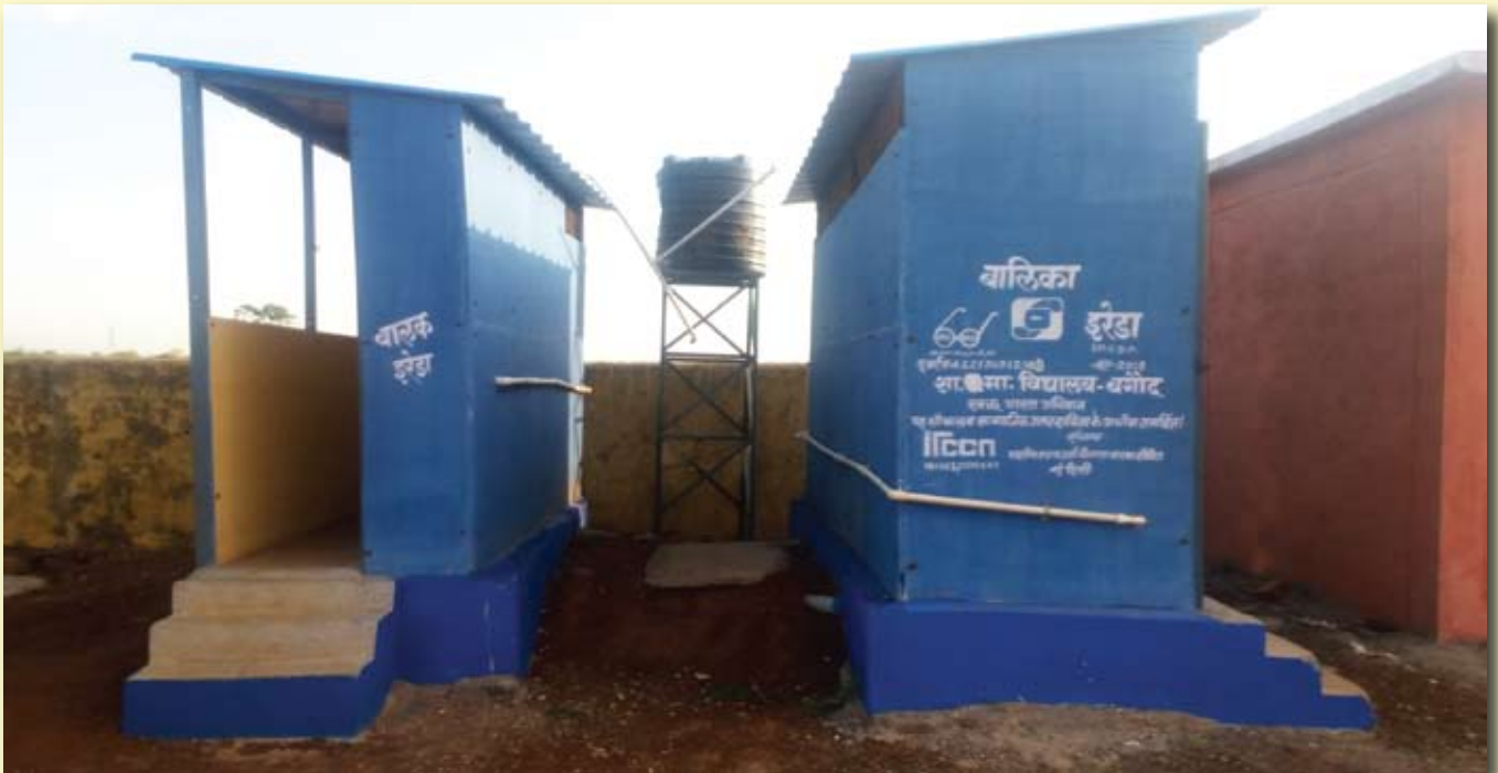
IREDA constructed toilets under the Swachh Bharat Mission of the Government of India.
