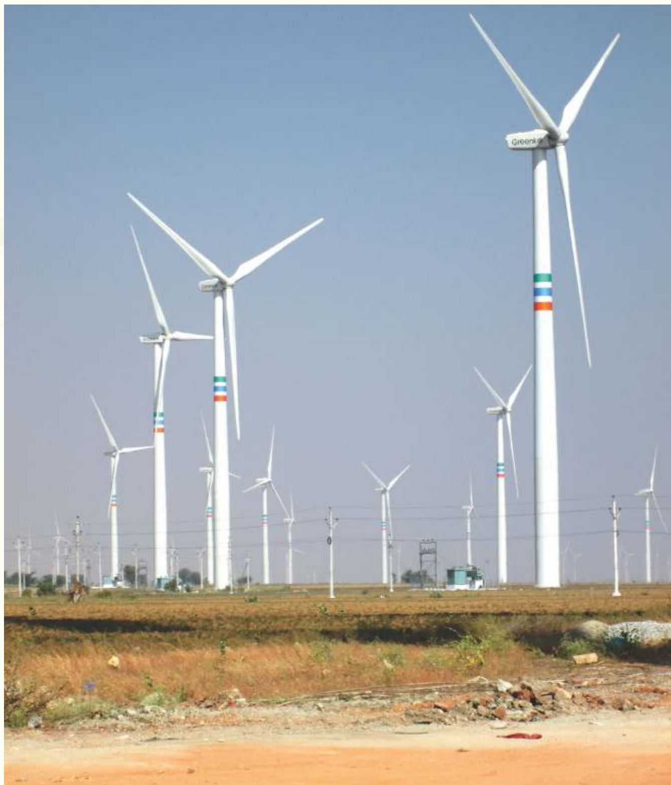
101.2 MW Wind Farm Project of M/s. Rayala Wind Power Company Private Limited (in Co-Financing Mode) Set up in Balavenkatapurum Village, Atmakur Taluk, Anantapur District of Andhra Pradesh
