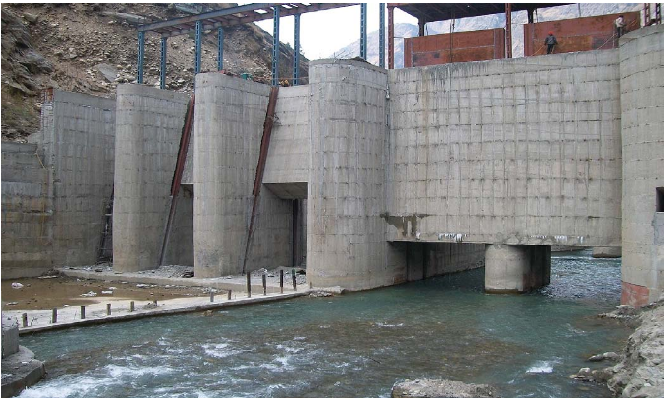
IREDA funded 13.2 MW SHP Project in State of Uttarakhand
