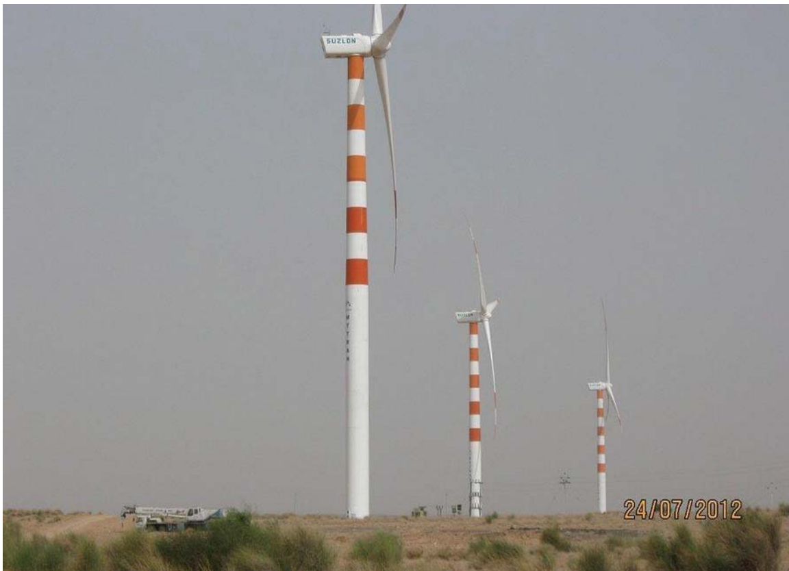
IREDA funded 232.2 MW wind power project at Rajasthan, Gujarat, Maharashtra & Karnataka.
