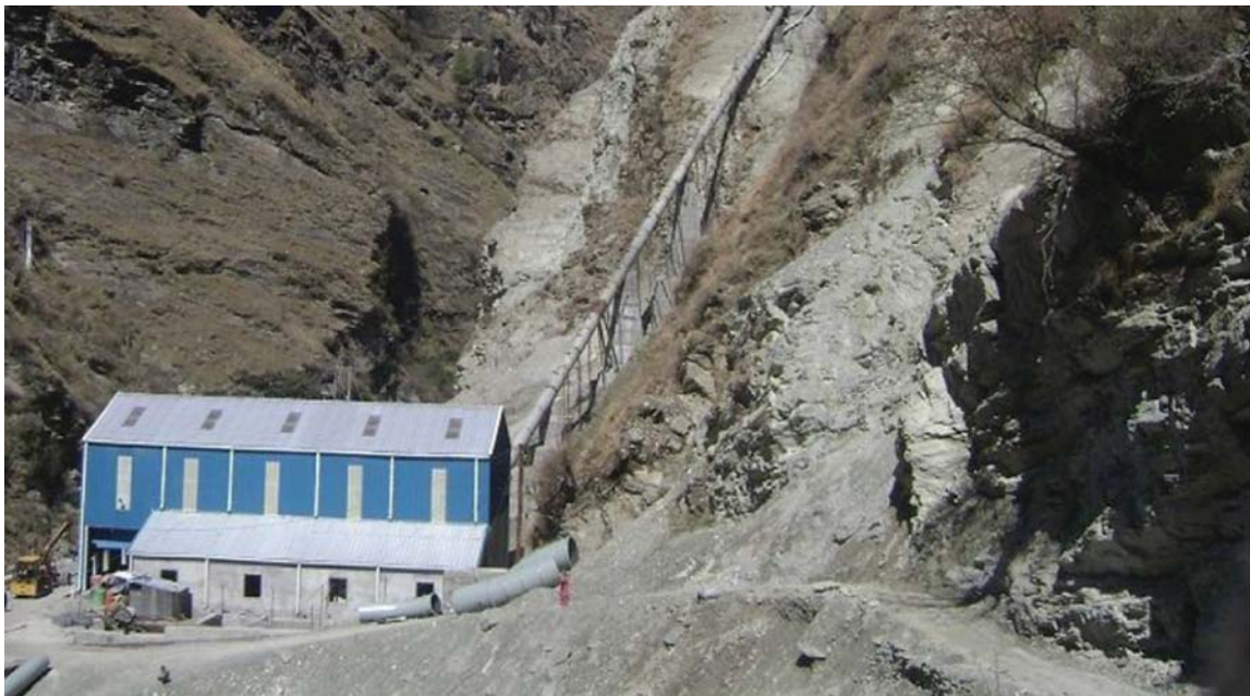
IREDA funded 5 MW Tarela-III in State of Himachal Pradesh
