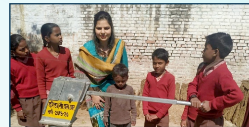
100 India mark II hand pumps were installed in rural areas of Machhlishahr, UP
