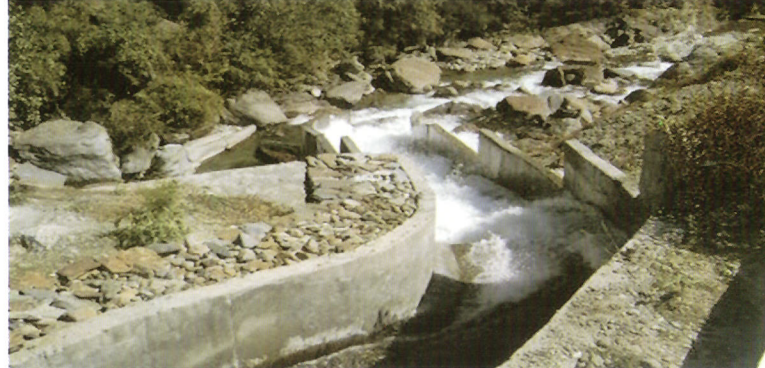
View of Tailrace
