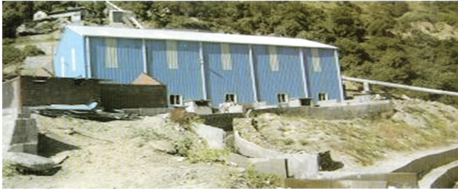
View of Power House
