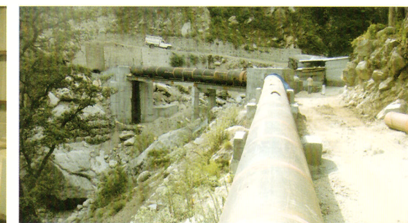
View of Power Channel
