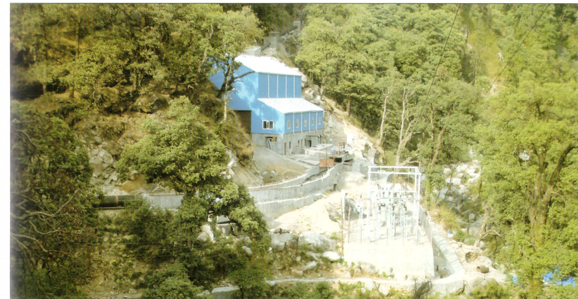
View of Power House &amp; Switchyard
