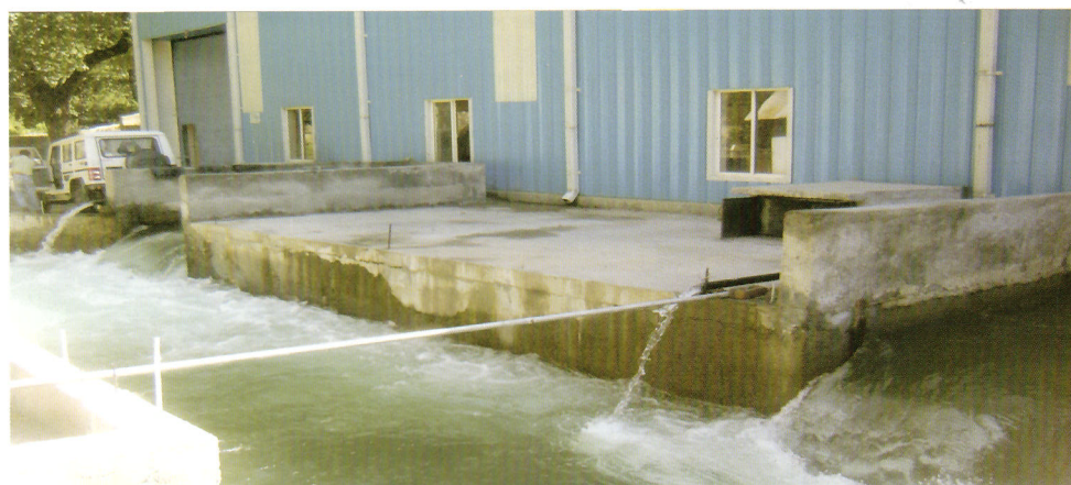
View of Power House &amp; Switchyard and Tailrace of IREDA funded 5 MW Taraila -II SHP project at Chamba District, Himachal Pradesh
