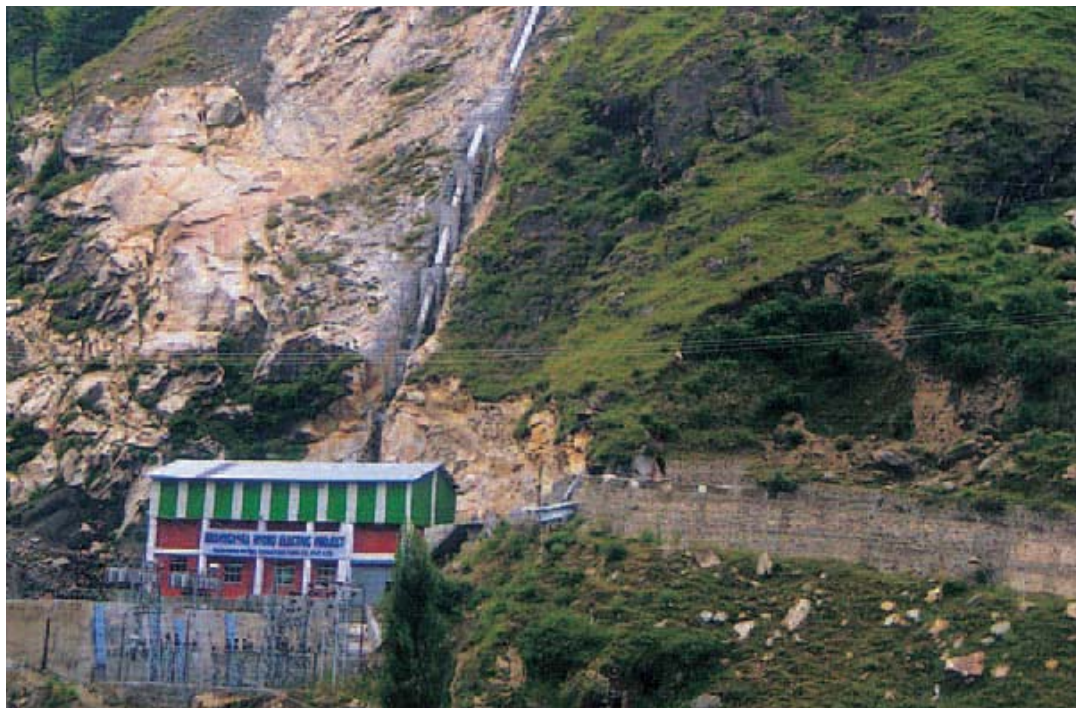
IREDA financed 5 MW Brahmaganga Small Hydro Project at Kullu District, Himachal Pradesh.
