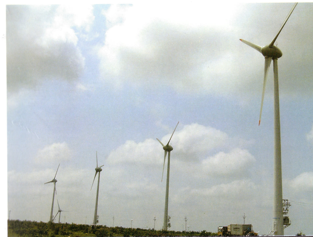
IREDA financed Windfarm Project at Dewas, Madhya Pradesh
