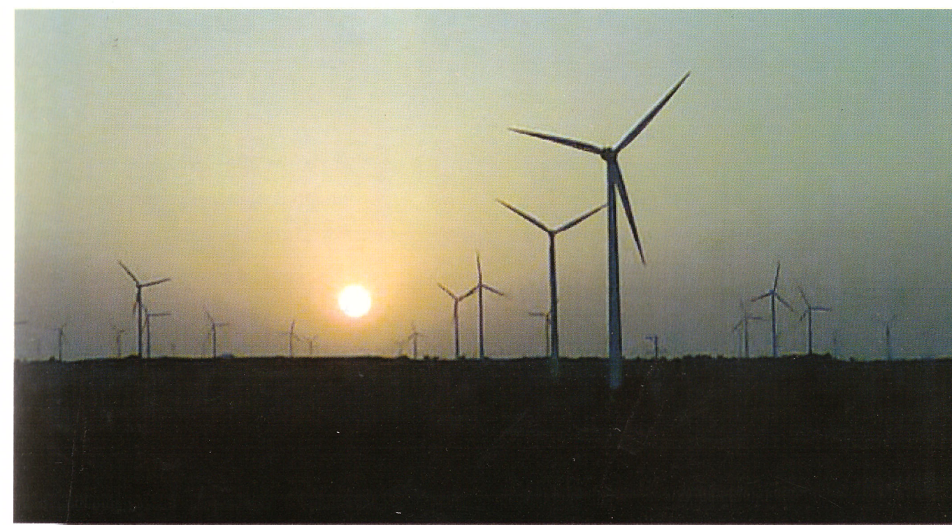
IREDA financed Windfarm Project at Jaisalmer, Rajasthan
