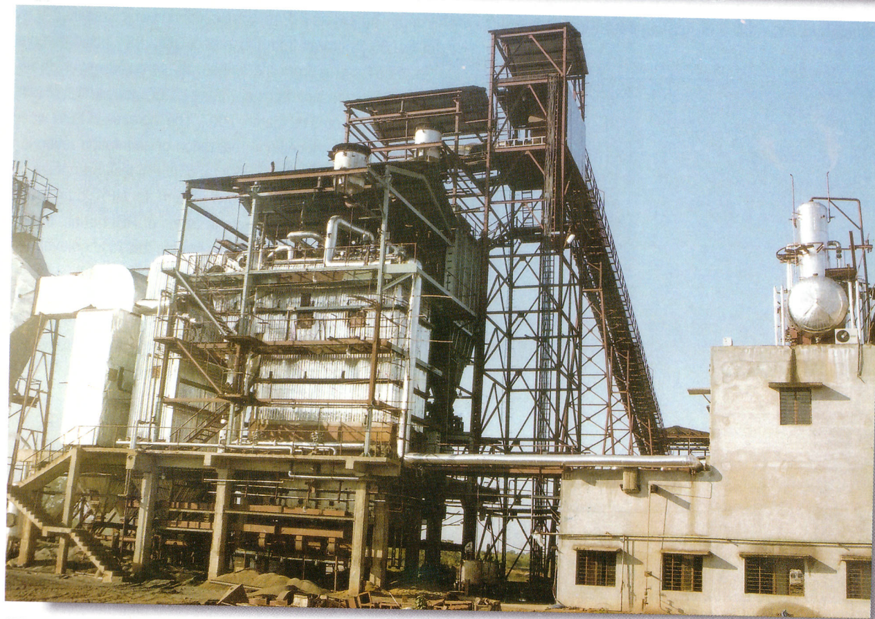
IREDA financed 7.50 MW Biomass Power Plant set up at Simga Village, Raipur District, Chhattisgarh.
