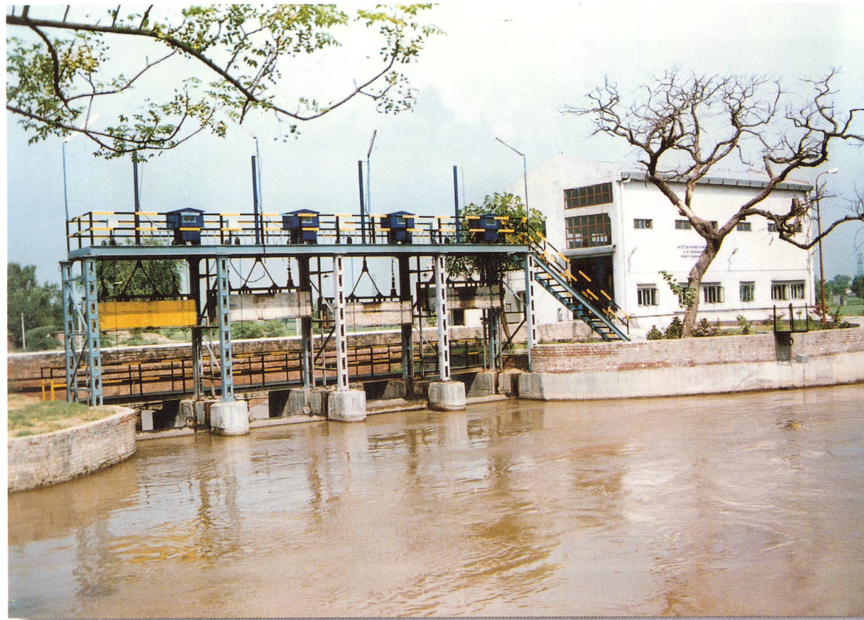
IREDA financed 1 MW Small Hydro Project set up at Sangrur District, Punjab under World Bank Line of Credit.
