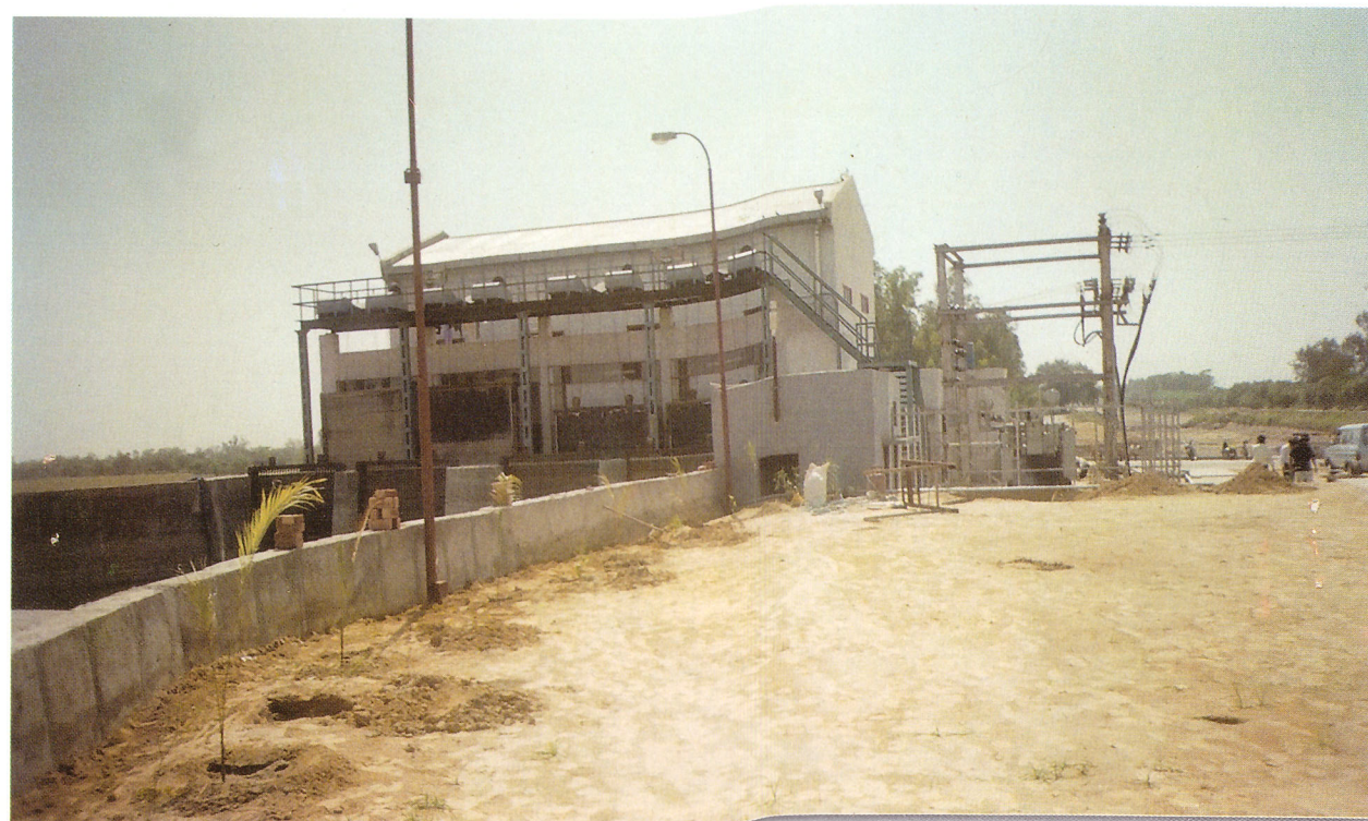
A view of IREDA financed 1.75 MW Small Hydro Project set up at Sangrur District, Punjab under World Bank Line of Credit.
