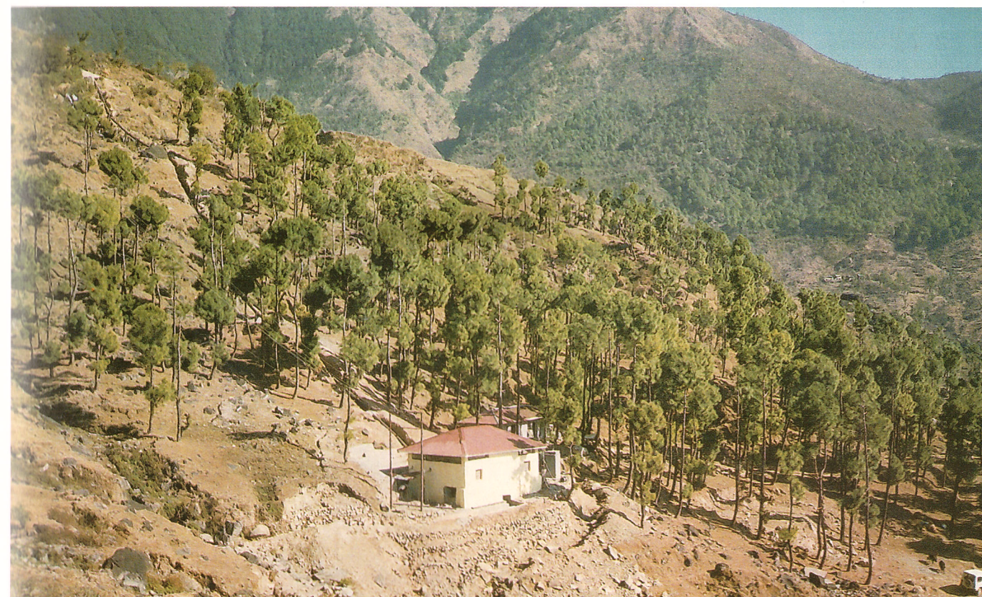
A view of head race channel bringing water to the penstock and power house of IREDA financed 0.15 MW Small Hydro Project set up at Hamirpur District, Himachal Pradesh under World Bank Line of Credit.
