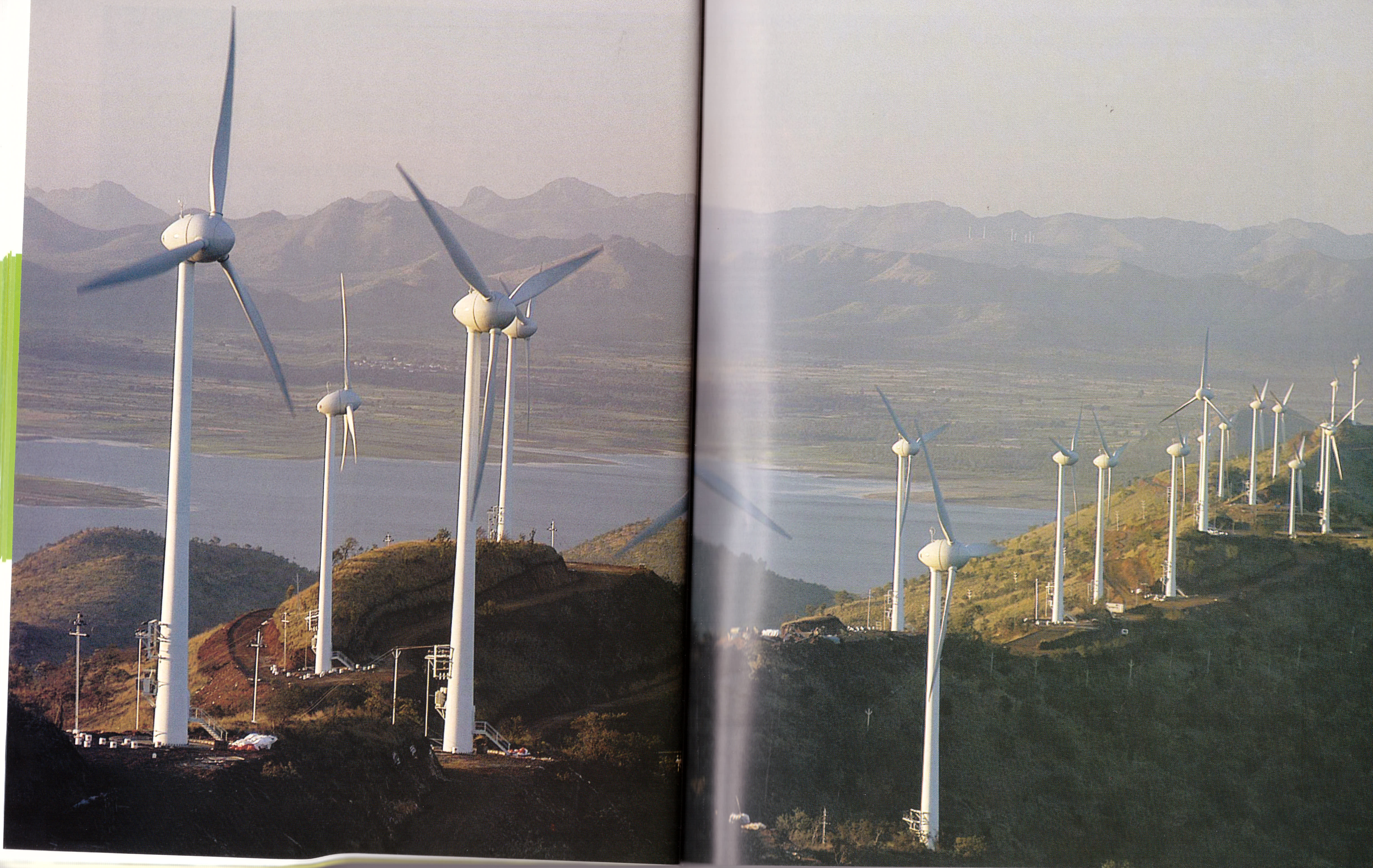
IREDA financed 4.2 MW Wind Farm project set up in Chitradurga District, Karnataka.
