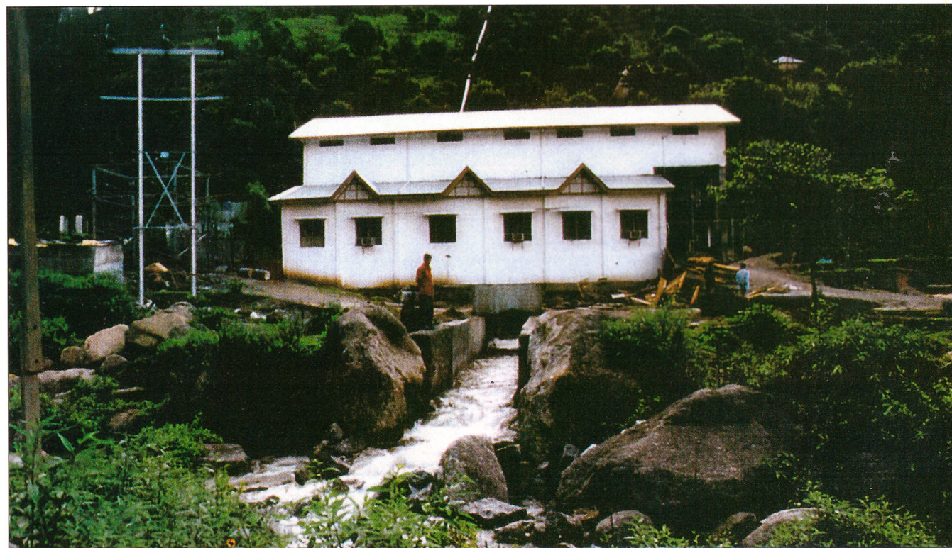
IREDA financed 5 MW Dehar Small Hydro Power project set up in Chamba District, Himachal Pradesh under Word Line of Credit.
