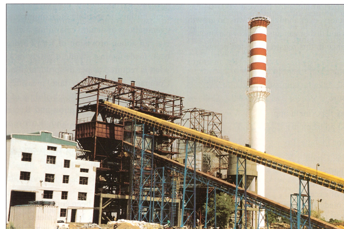
IREDA financed 6 MW Biomass power project set up at Gudebelluru Village, Maganur Mandal, Mahabubnagar District, Andhra Pradesh.
