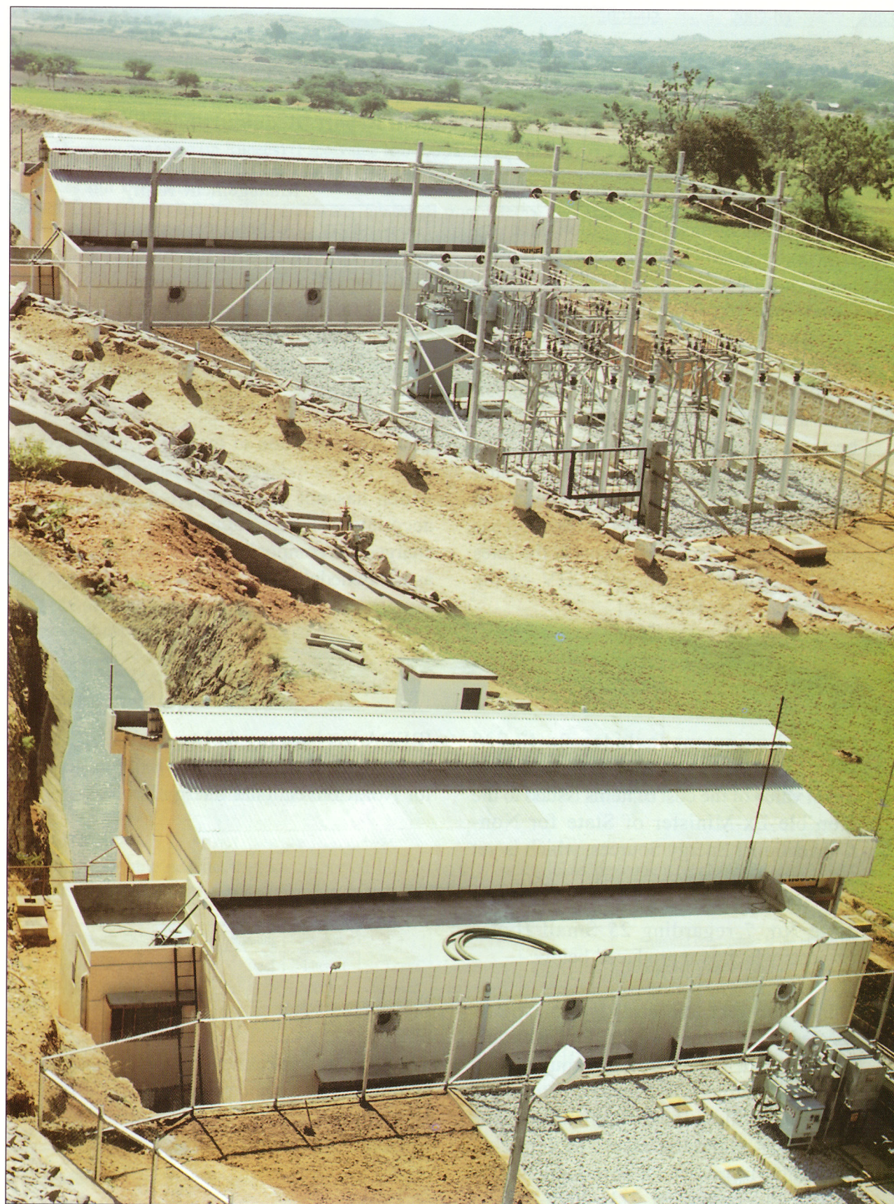
IREDA financed 0.8 MW SHP project set up at Banathal Village, Gulbarga District, Karnataka under World Bank line of credit.
