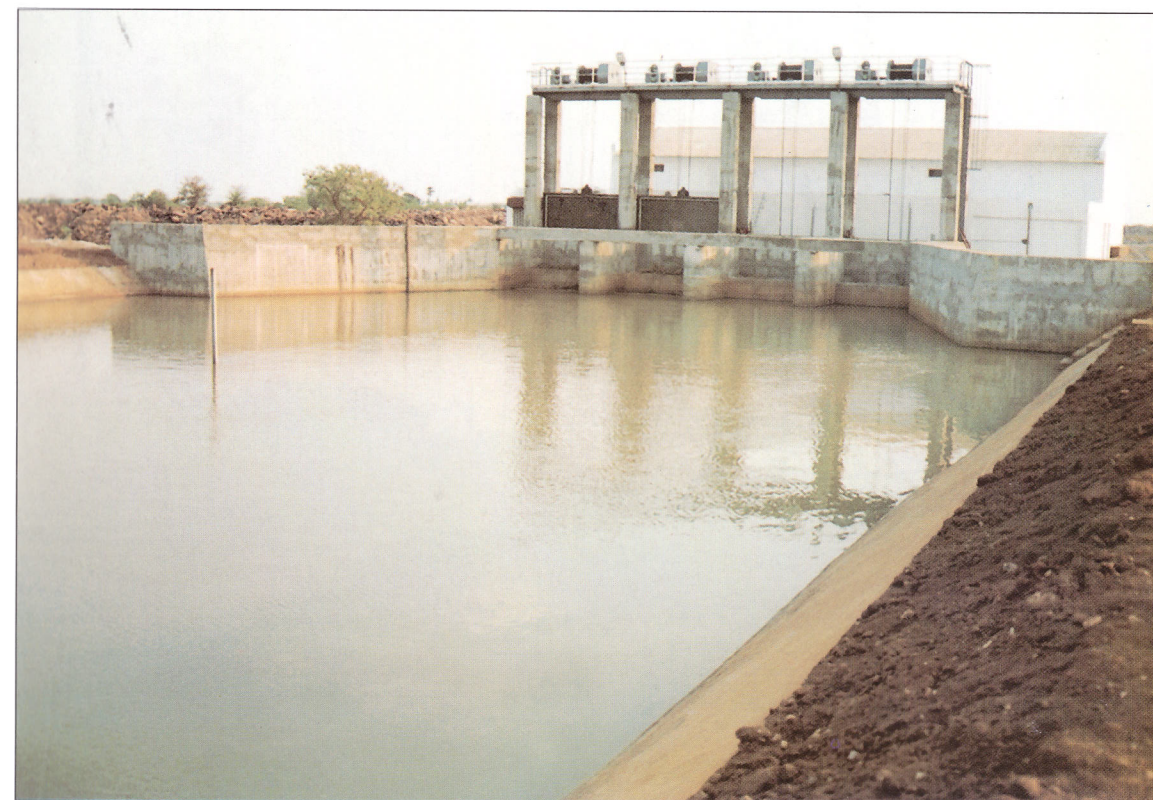
In take structure & power canal view of IREDA financed 4.00 MW Small Hydro project set up at Madhavaram District, Andhra Pradesh.
