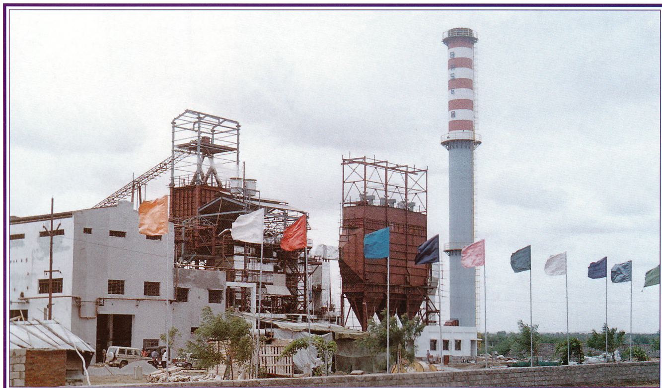
IREDA financed 6 MW Biomass Power Project under implementation at Hegasnahalli village, Deosugurhobli Taluka, Raichur District, Karnataka.
