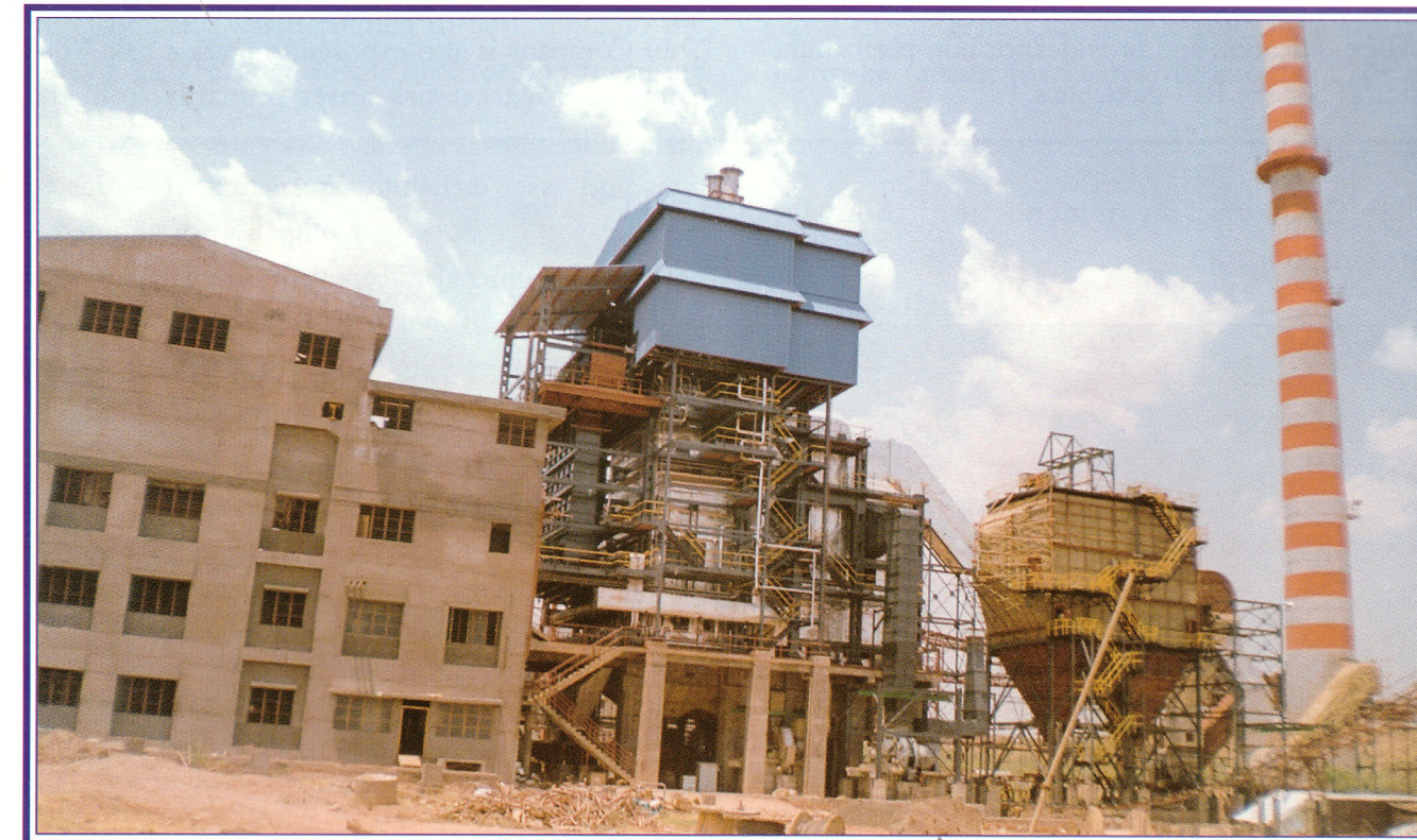
IREDA financed 22.5 MW Bagasse based Co-generation project set up at Bagalkot District, Karnataka.
