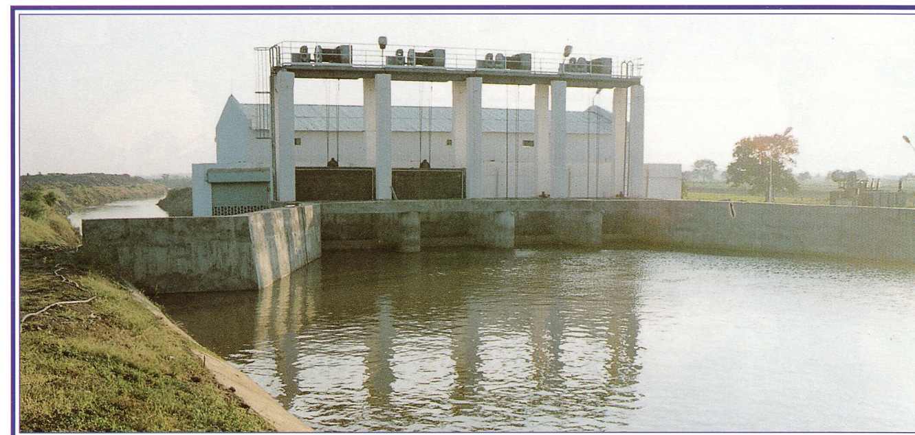
IREDA financed 3.30 MW Small Hydro Power project set up at Village Velpanur, Kurnool District, Andhra Pradesh under the World Bank Line of Credit.
