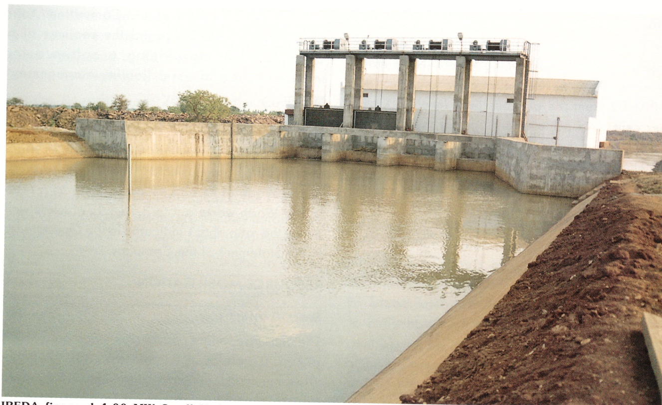
IREDA financed 4.00 MW Small Hydro Project set up at Nippulavagu, Guntakandala Village, Kurnool District, Andhra Pradesh under the World Bank Line of Credit.
