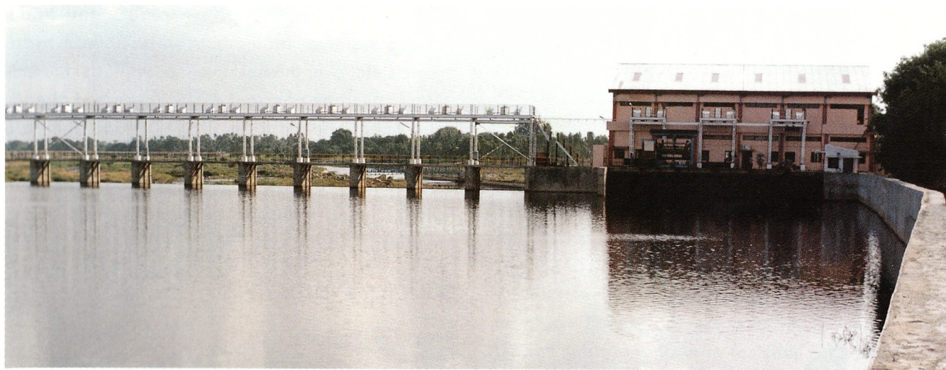
IREDA financed 3 MW Small Hydro Project set up at Madhavamanthri Dam, Mysore District, Karnataka under the World Bank Line of Credit.
