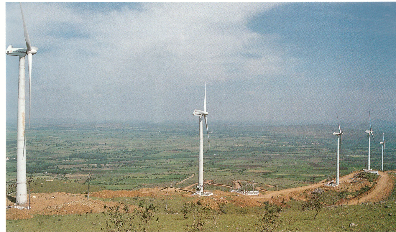
IREDA financed 3.75 MW Wind Farm set up at Bidrekere Ridge, Davengere District, Karnataka.
