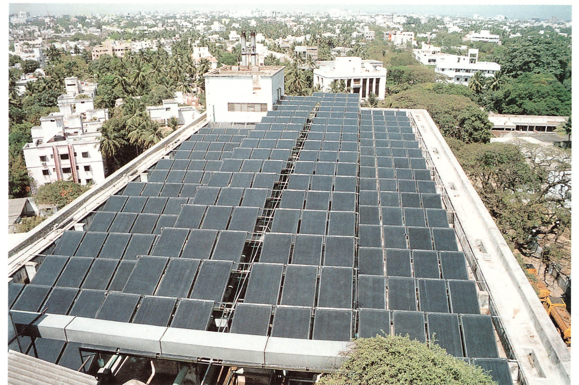
IREDA financed 42000 LPD Solar Water Heating System installed on the roof of a five star hotel in Chennai, Tamilnadu.
