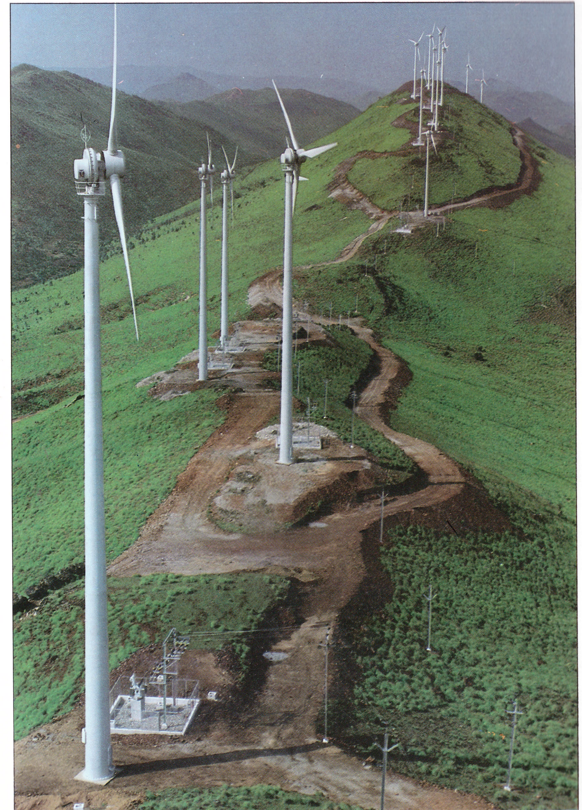
IREDA financed 7.59 MW Wind Farm Project set up in Chitradurga district of Karnataka.
