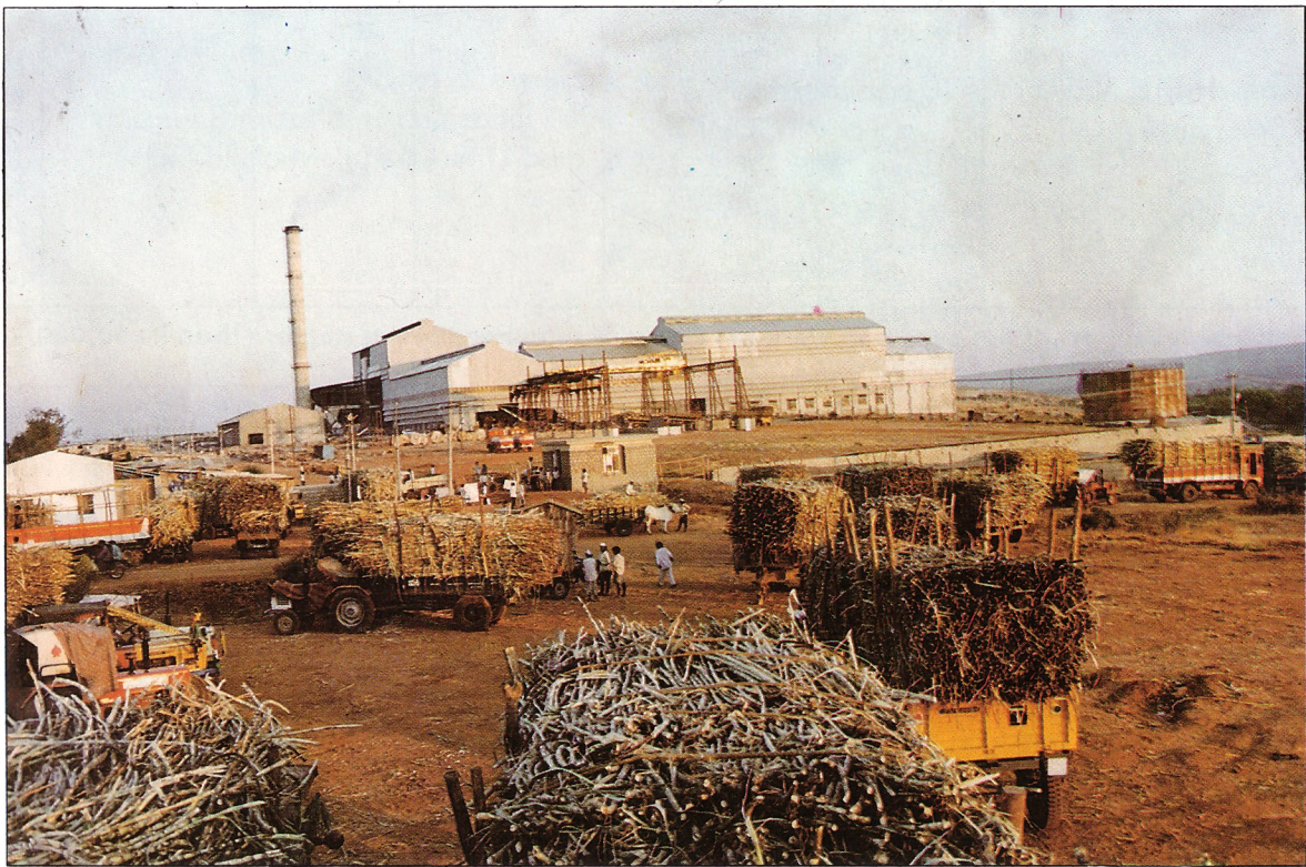
IREDA financed 11.2 MW Co-generation Plant Set up at Village Munoli, Belgaum district, Karnataka.
