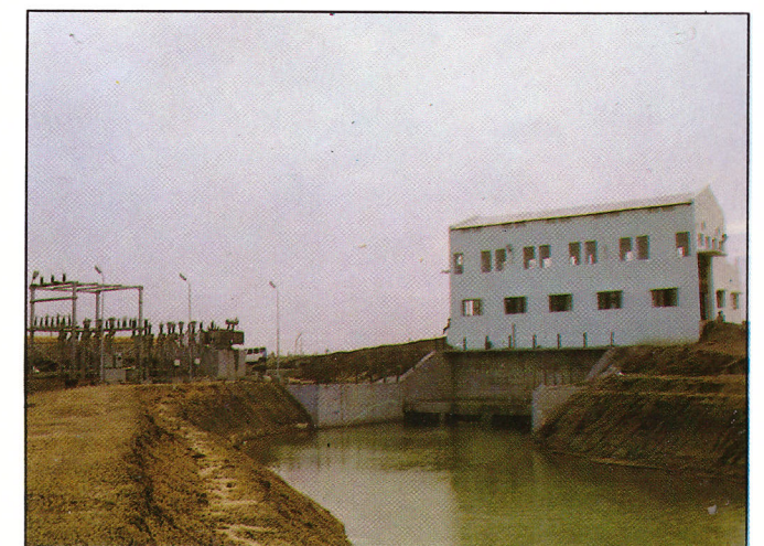
Mini Hydel Power House project set up near Sattenapalli, Guntur District, Andhra Pradesh financed by IREDA under World Bank Line of Credit.
