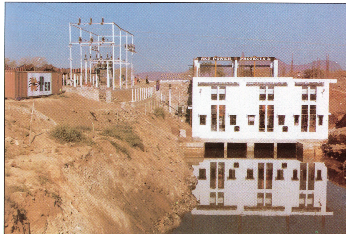
IREDA financed 1.5 MW Small Hydro Project set up at Ongole branch canal, Darsi Village, Prakasam District, Andhra Pradesh, under the World Bank Programme.
