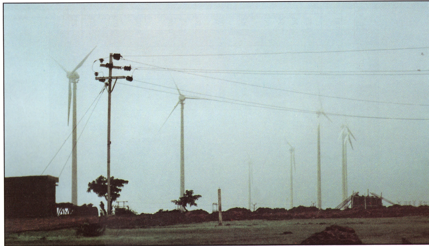
IREDA financed 3.91 MW Wind Farm project set up in Satara District, Maharashtra.
