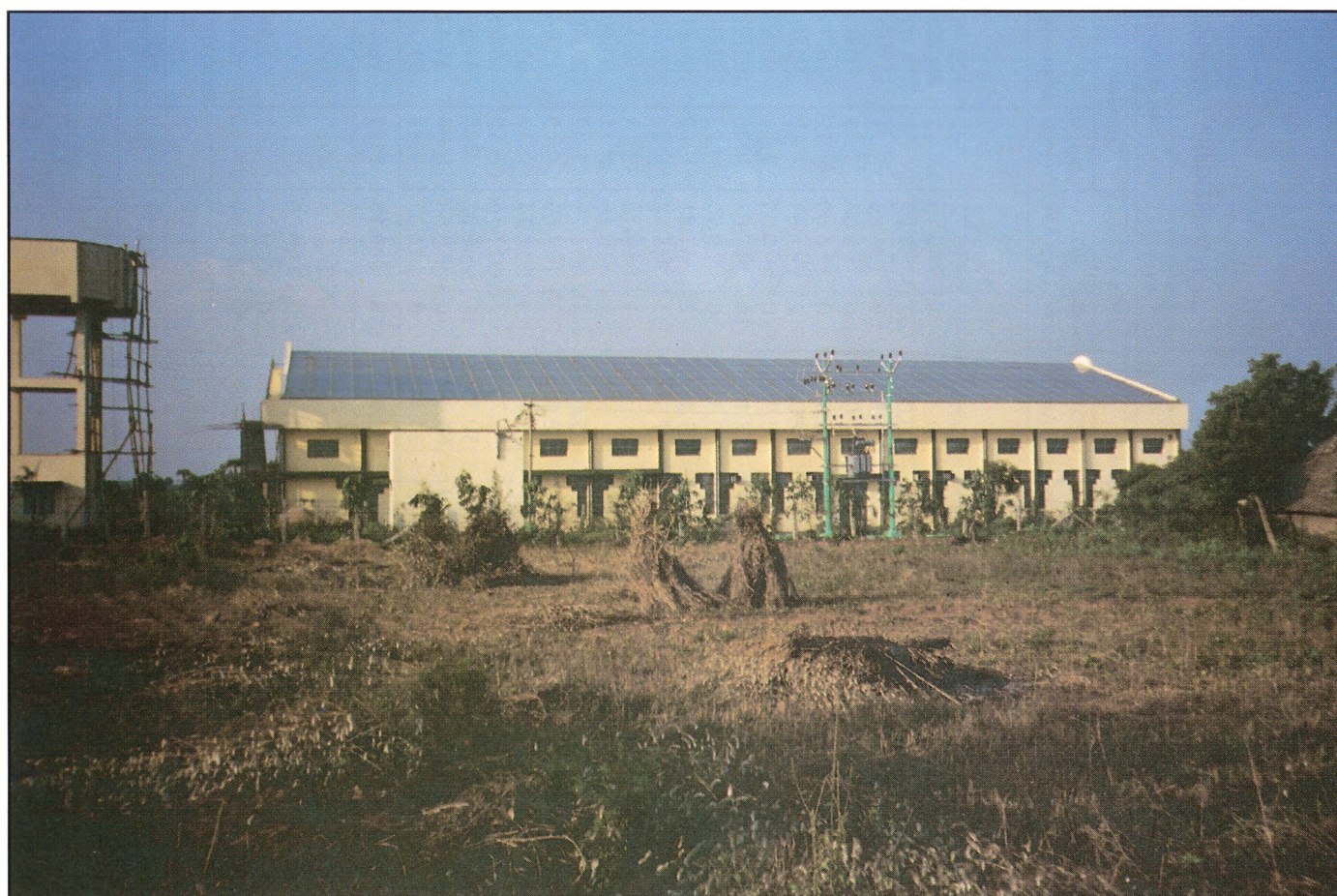
IREDA financed 600 sq. mtr. Solar Air Heating System for drying of spices installed in Erode, Tamilnadu.
