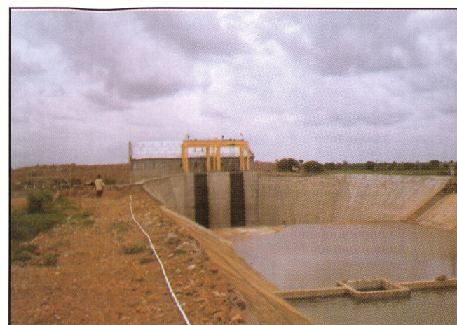
4.0 MW Small Hydro Project set up in Atmakur Village, Kurnool District of Andhra Pradesh, under World Bank Programme through IREDA.
