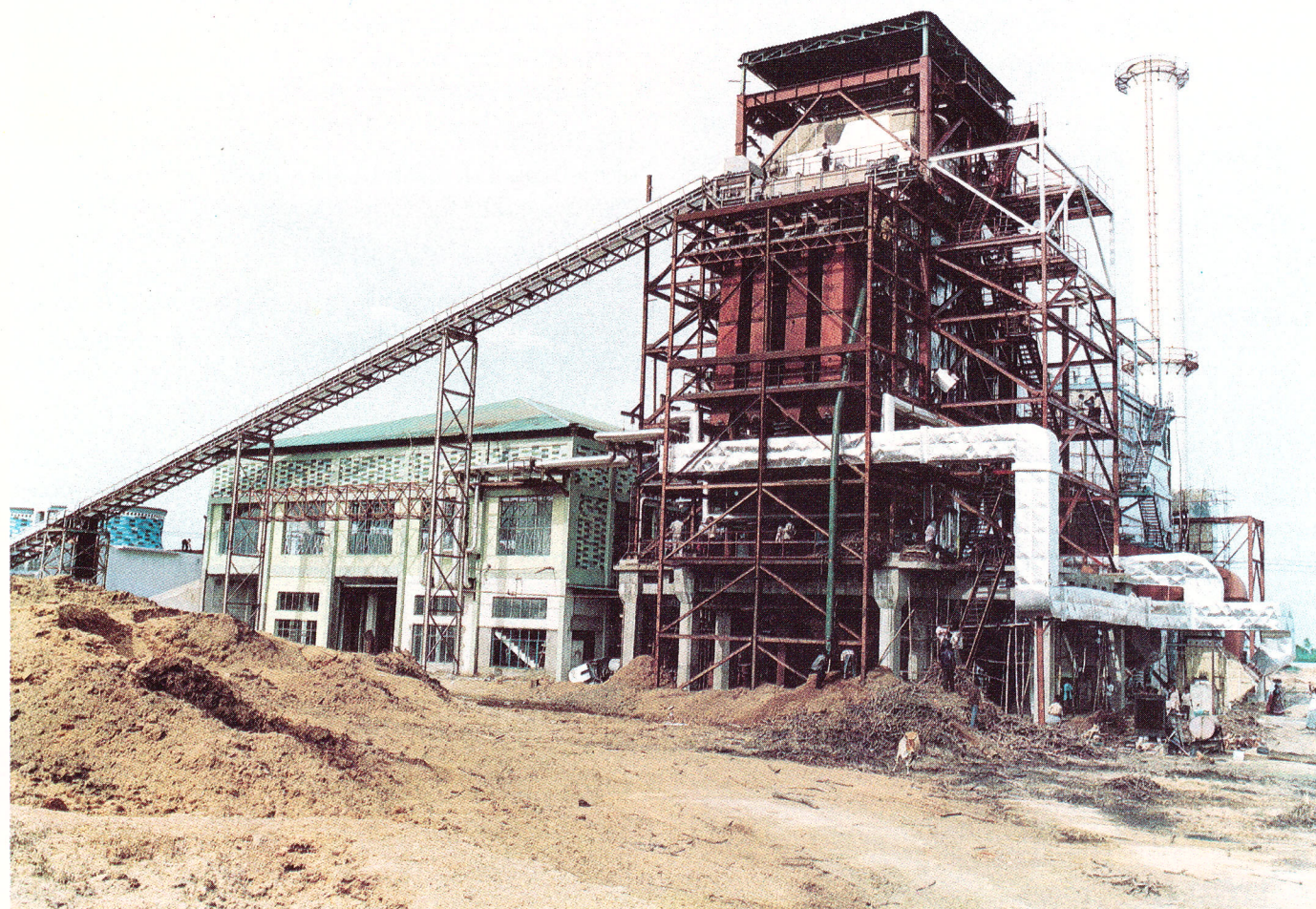
IREDA financed 12 MW Biomass Power Plant set up in the State of Tamilnadu.
