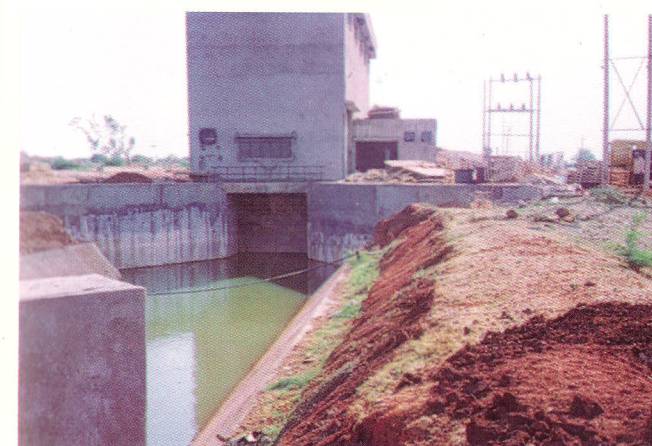
1.3 MW Irrigation Canal based Mini Hydel Project set up with IREDA's assistance under the World Bank Line of Credit in Karnataka State.
