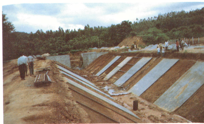
A view of 'canal lining panel casting' of 1.5 MW Small Hydro Project funded by IREDA from World Bank funds under the "India: Renewable Resources Development Project" at Shimoga district of Karnataka.
