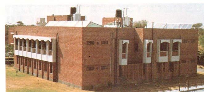
14,200 LPD Solar Water Heating System installed with IREDA's assistance at a school in Bhiwani, Haryana
