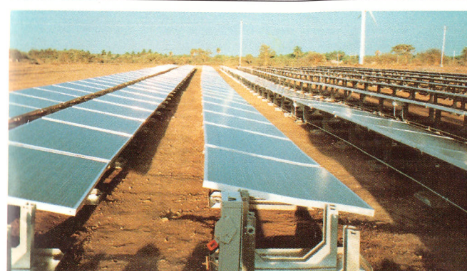
100 KW Grid connected SPV Power Plant set up in the existing wind farm in Tamil Nadu, financed by IREDA under the 'SPV Market Development Programme' of World Bank.
