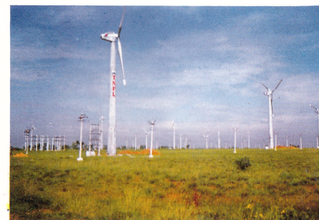
A 15 MW wind farm project set up in the State of Tamil Nadu with assistance received from the World Bank under INDIA: Renewable Resources Development Project by IREDA.
