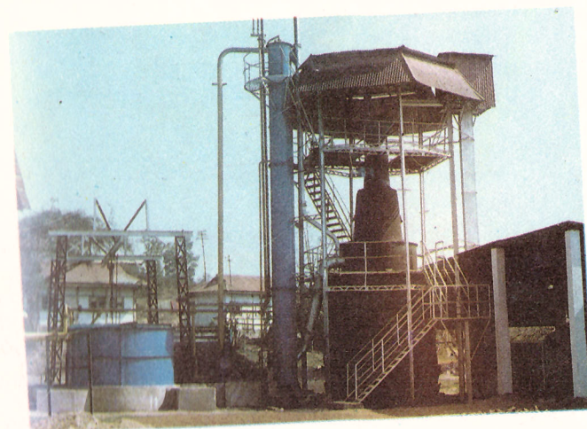
Paddy based husk gasification plant developed by an institution supported by IREDA.
